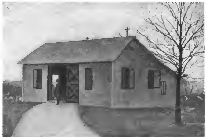
Garage in Cement, Combining Living Rooms
